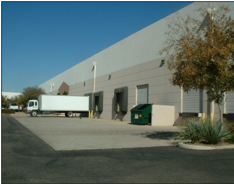
Unfavorable: Loading docks oriented towards street with unscreened refuse enclosure
