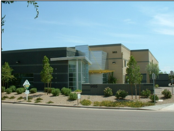
Favorable: Building design using forms and shapes to break up building mass
