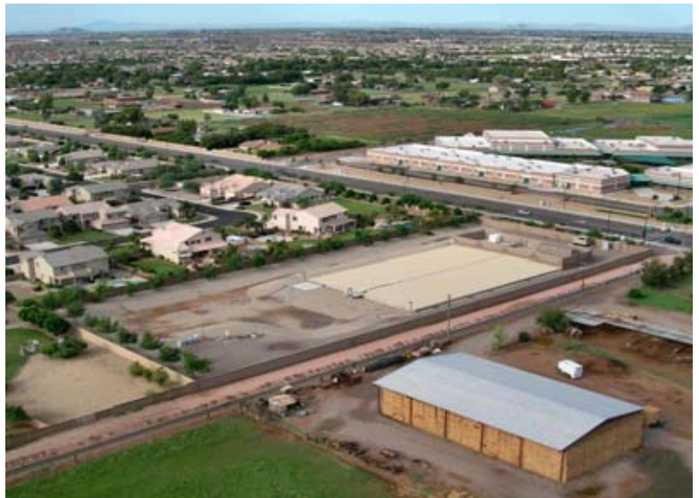
4 Million Gallon (MG) Reservoir - Lindsay Road
