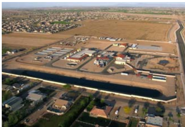
Santan Vista Water Treatment Plant
