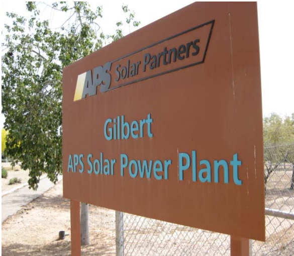
Gilbert APS Solar Power Plant
